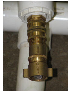
Hose Fitting Attached (Note Directional Arrow)
